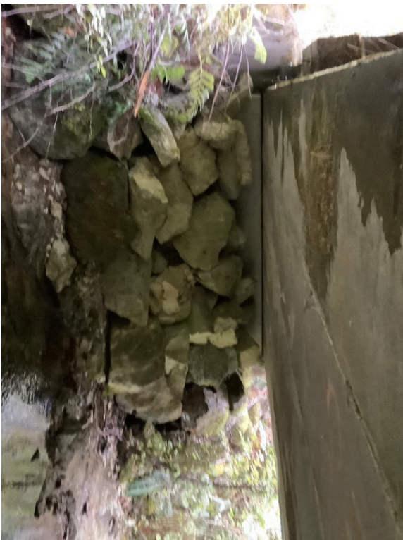
Left Bank Abutment when facing downstream
