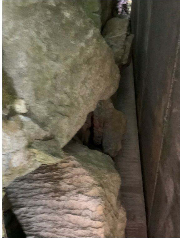
Right Bank Abutment when facing downstream
